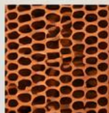
Perforated Brick Screen
